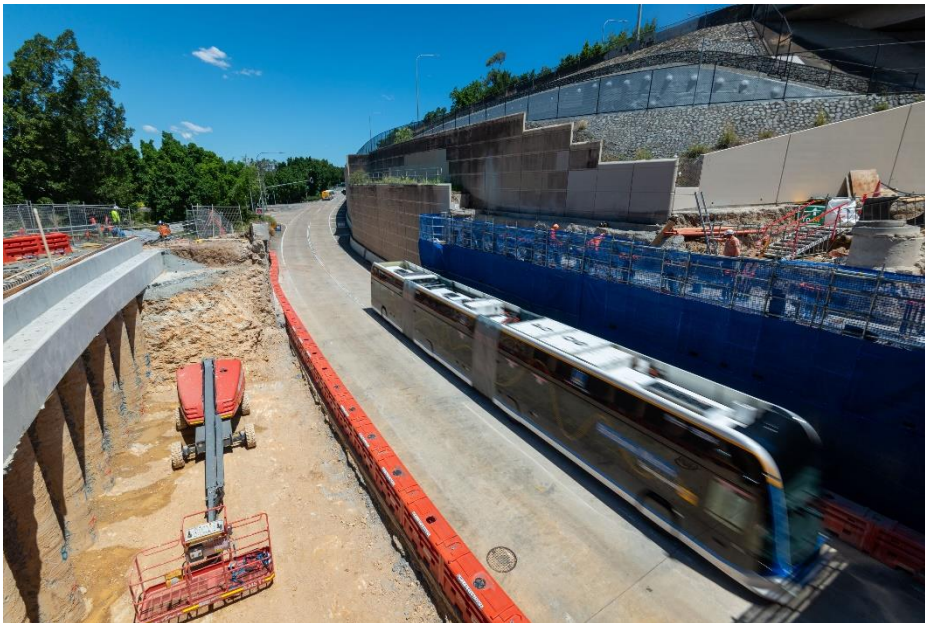
Image: Construction activities underway at Buranda busway station
