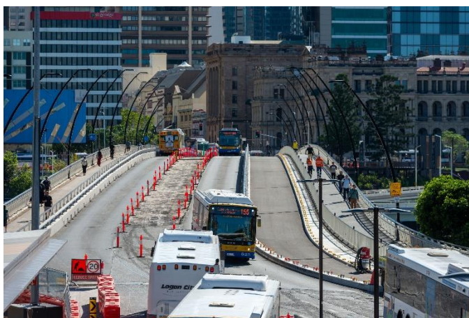
Image: Resurfacing works on Victoria Bridge
