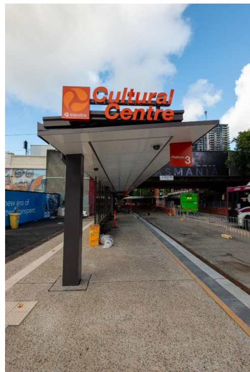
Image: Finishing works underway at Cultural Centre station.
