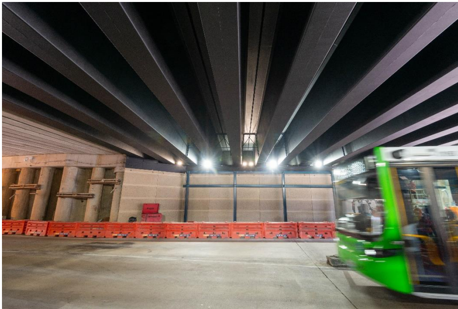
Image: Platform construction in progress.
