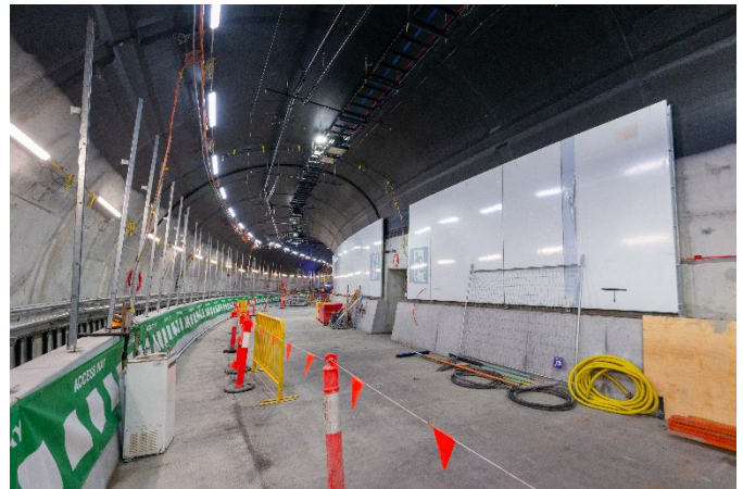
Image: installation of cladding within the Adelaide Street tunnel
